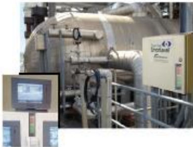
Eye-Hye® SmartLevel™ With Local and Remote Indicators
